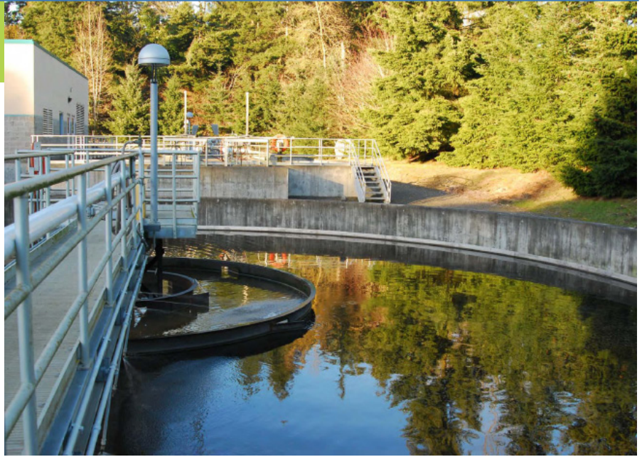
Built in 1971, Wilsonville's wastewater treatment plant is being upgraded to meet community needs and environmental regulations.
